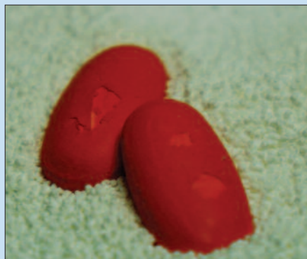
b. Peeling can occur when the initial coat isn't allowed to dry before additional coats are applied.
